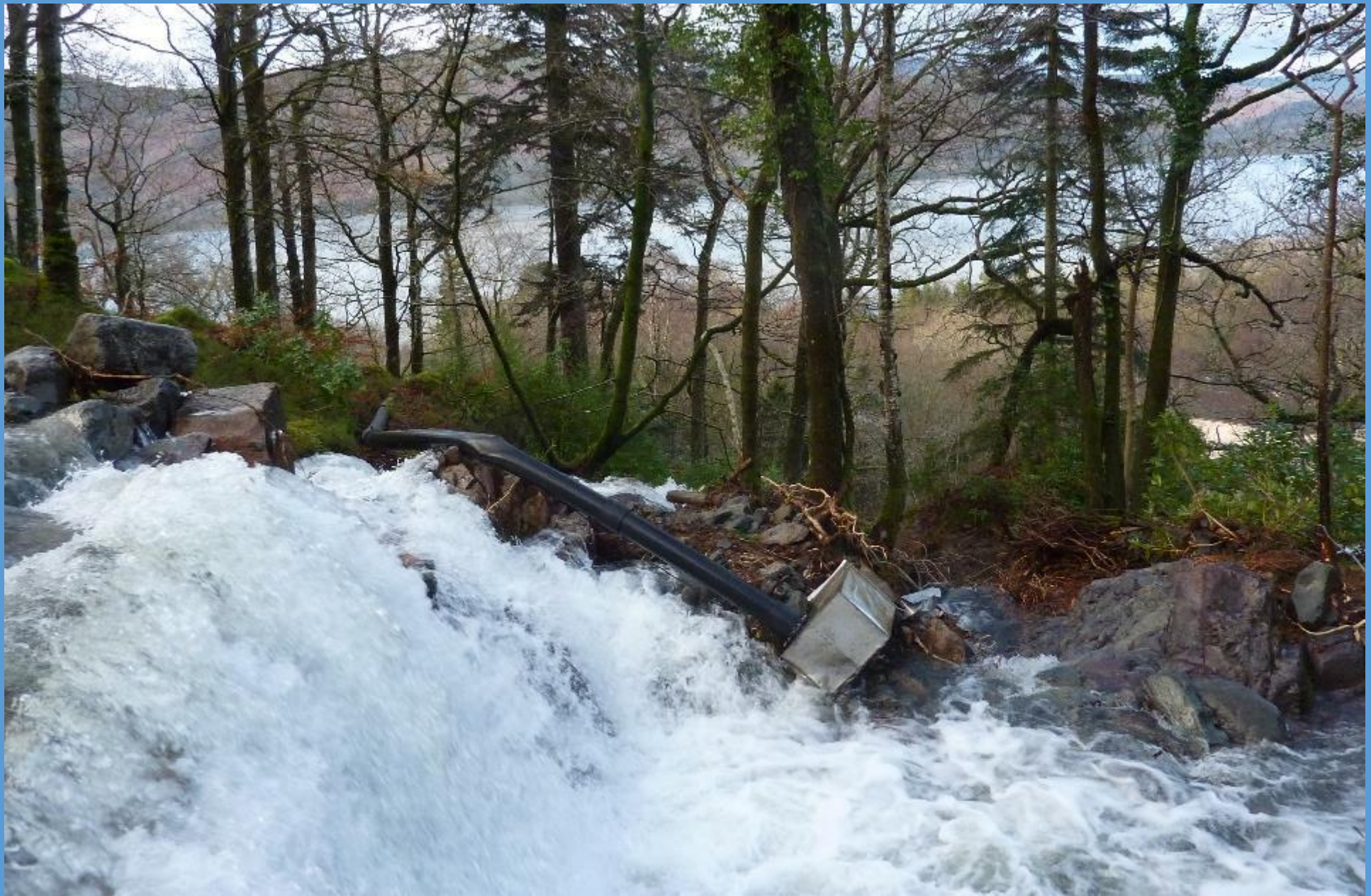
At the dam on Barrow Beck, parts of our hydro-electric plant were damaged. Here you can see the Forebay tank and the connecting pipe, which were wrenched away from the dam. The pipe usually delivers water to the turbine. So unfortunately we couldn't take advantage of the high volumes of water for electricity generation. Sun 6 th Dec.
