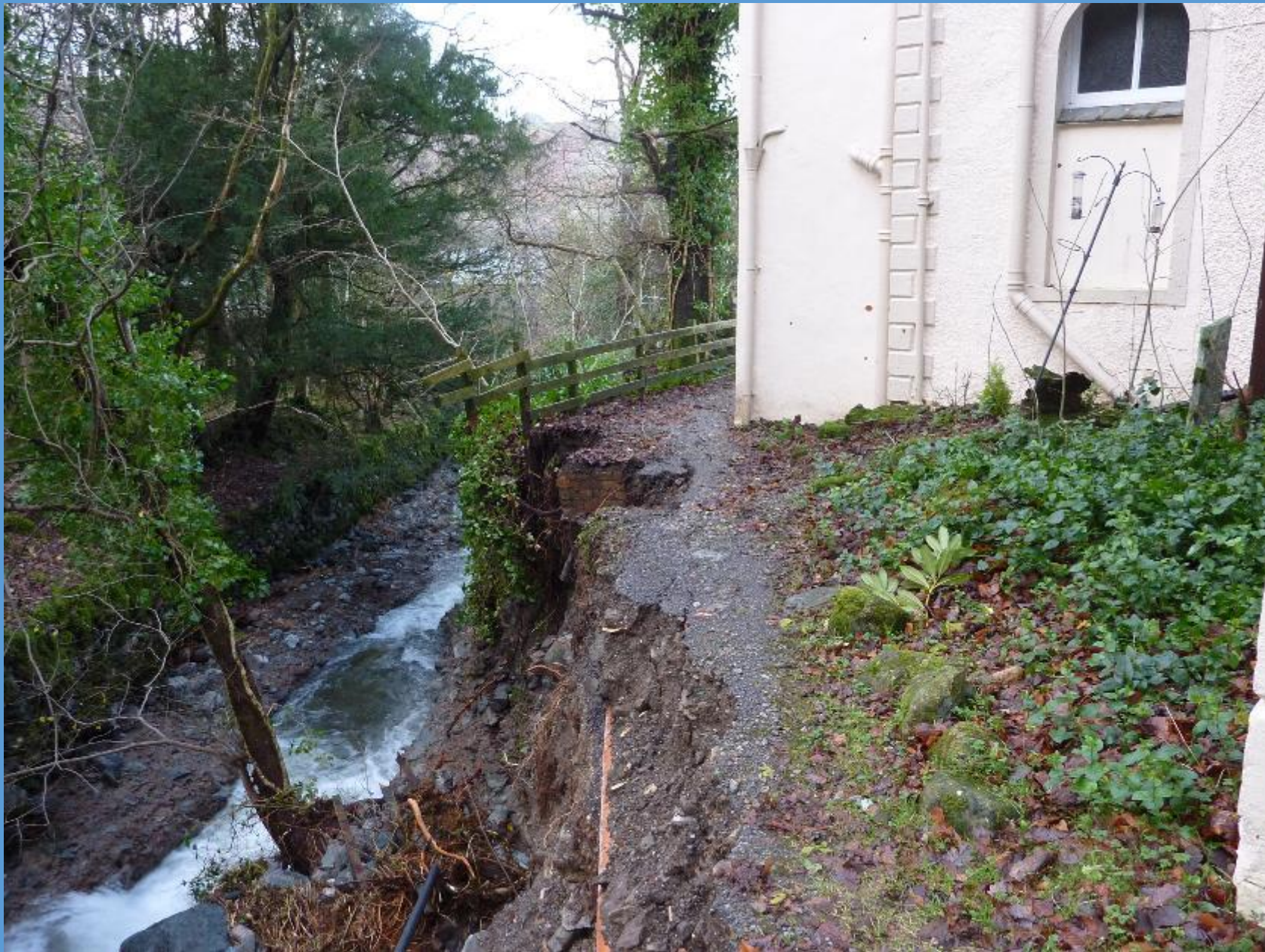
Looking at the rear of the hostel, where the footpath collapsed, damaging mains and waste pipes in the process. Luckily the foundations of the house were not damaged. Mon 7 th Dec.
