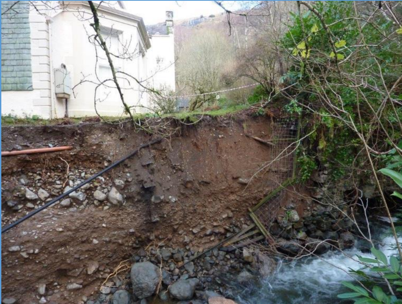
A view from the beck channel, where the mains water and waste pipes run through the banks. Mon 7 th Dec.
