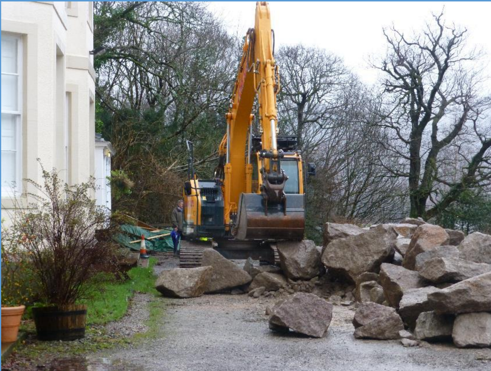
The diggers moved £40 000 worth of boulders into the channel of Barrow Beck, to re-inforce the banks.
